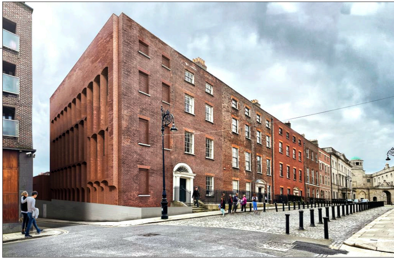
Artist's impression of the expanded headquarters of Na Píobairí Uilleann in Henrietta Street, Dublin.
